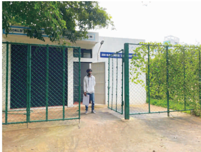
Sewage treatment plant
